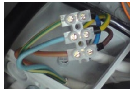
Fig. 7: Here N and PE have been reversed
